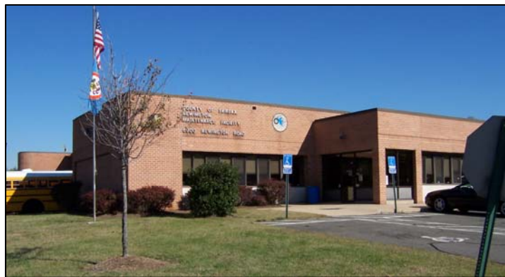
Picture of existing Newington facility
