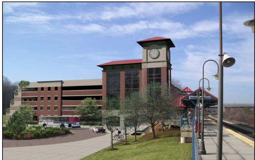
Burke Virginia Railway Express (VRE) Station.
