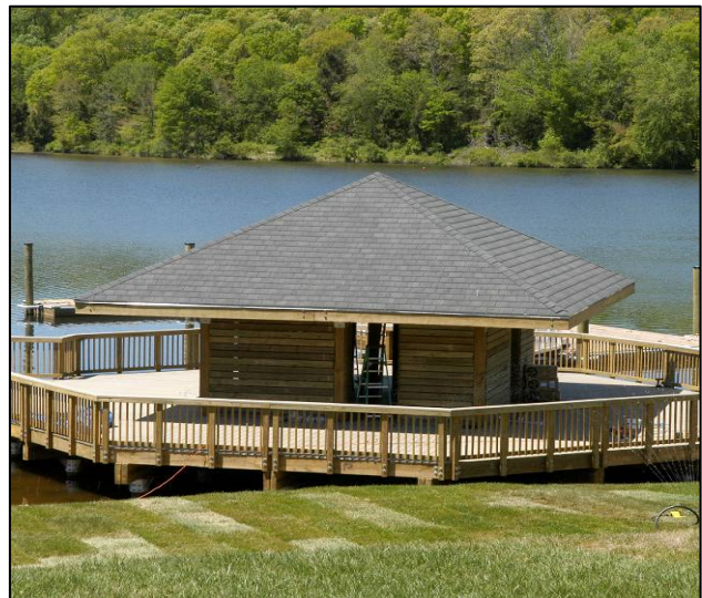
Picture of new dock at Lake Fairfax
