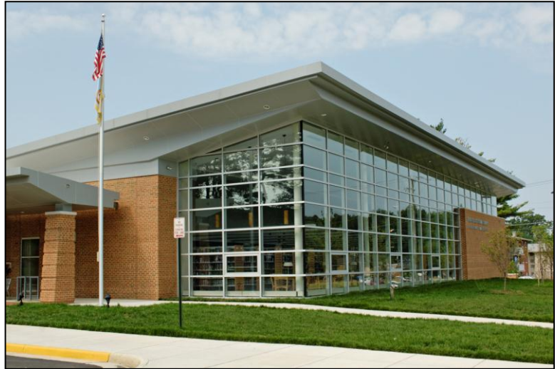
The renovation of the Thomas Jefferson Community Library, located in Falls Church, was completed in 2010. Photo credit: Paul Thornily.
