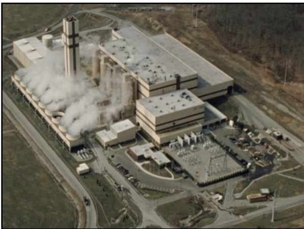
I-95 Energy/Resource Recovery Facility
