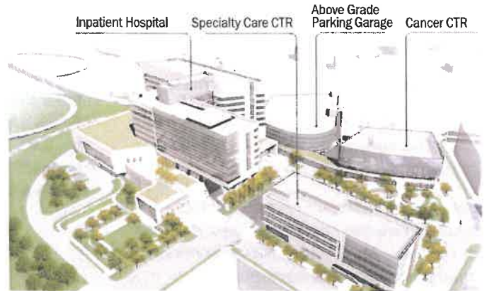
Inova Health Medical Campus under construction
