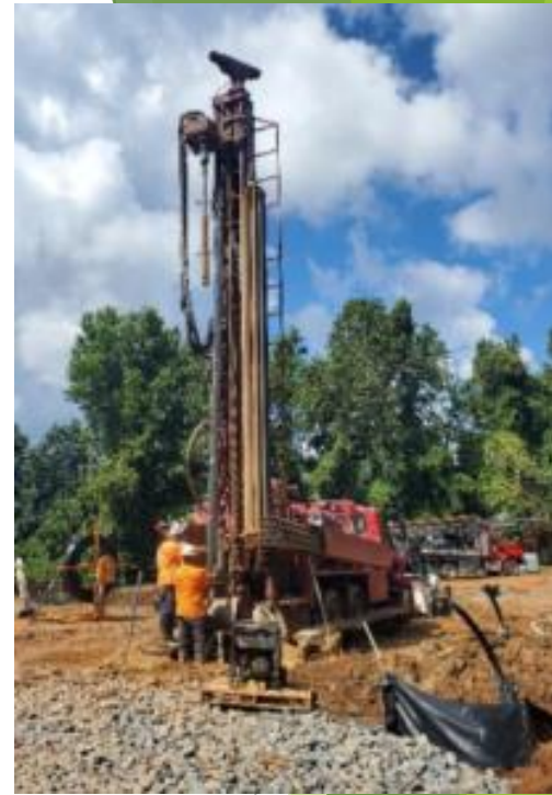
Spring Hill Rec Center Geothermal Wellfield (top) Rooftop Solar (bottom)
