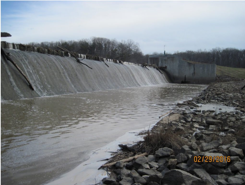
5. Looking northeast at the dam of Lake Accotink.
