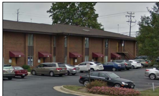
Office units in the Stuart Professional Village along Laurel Way
