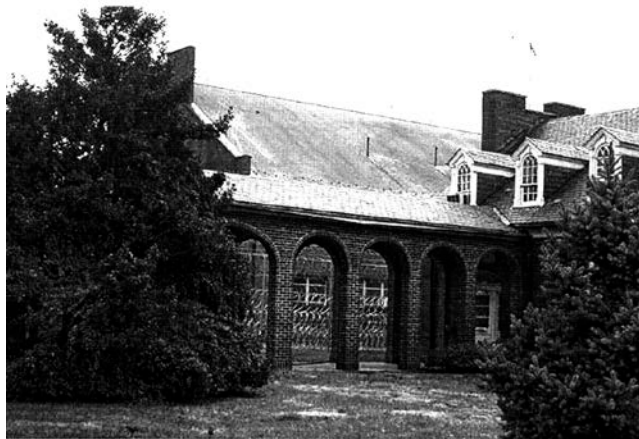
VIEW FROM ROUTE 123 OF THE ADMINISTRATIVE BUILDING AND THE OCCOQUAN FACILITY
