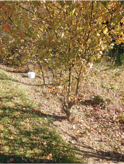
VEGETATED SWALE. Swale channel, plantings and observation well.
