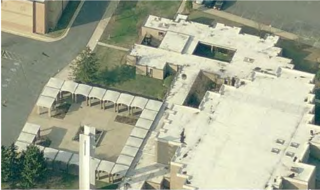
FM9500_1.jpg: View of open areas in front of church to site bioretention filters
