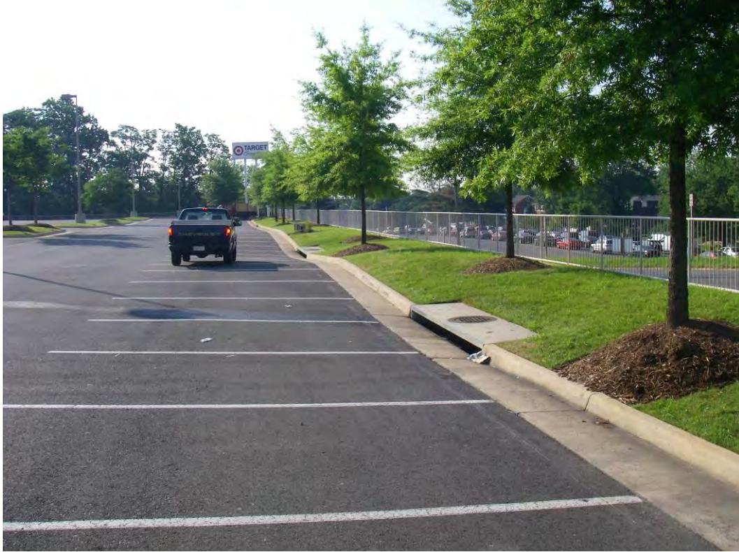
FM9503_1.jpg: View of existing inlet in parking lot
