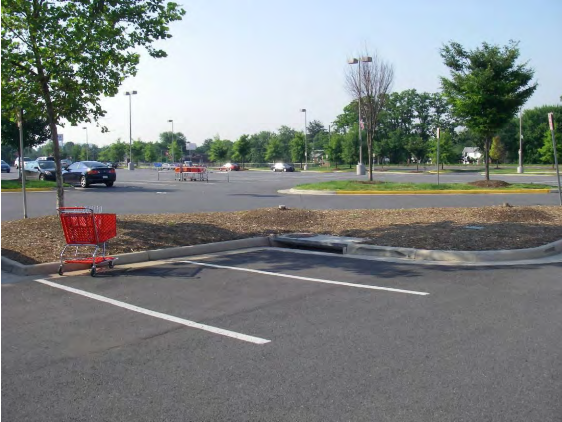
FM9502_1.jpg: View of existing inlets in parking lot
