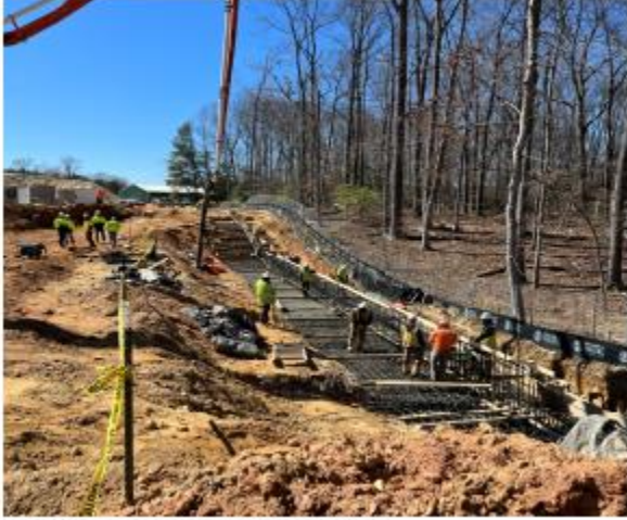
Pouring a stepped foundation
