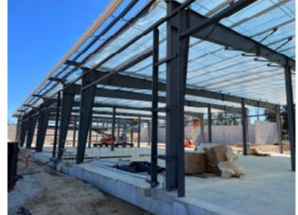
Continue framing PEMB structure, cleaning the slab
