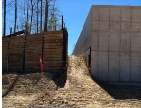
Backfilling soil and compacting
