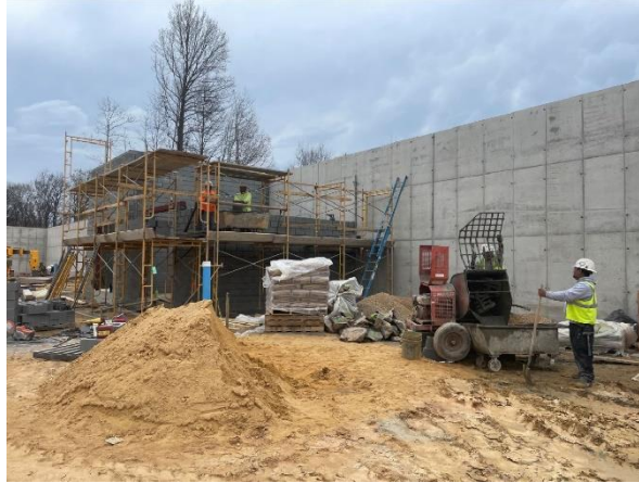
CMU wall with supporting steel
