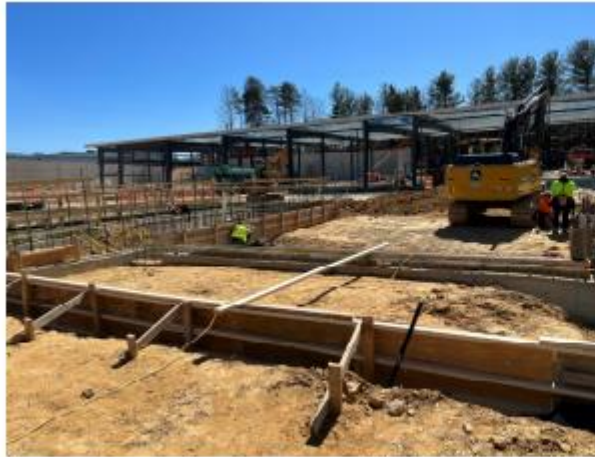
Concrete walls framing around Vector Decant area
