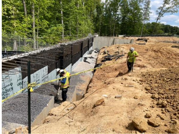
Damp proofing and foundation drains
