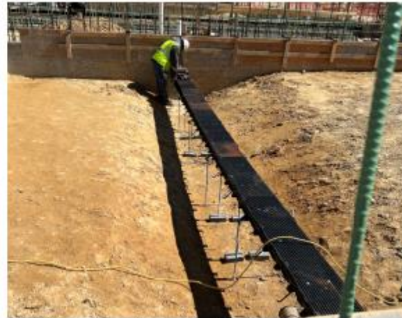
Installing trench drain in Vector decant
