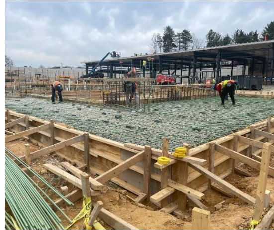
Steel reinforcement and gravel at slab
