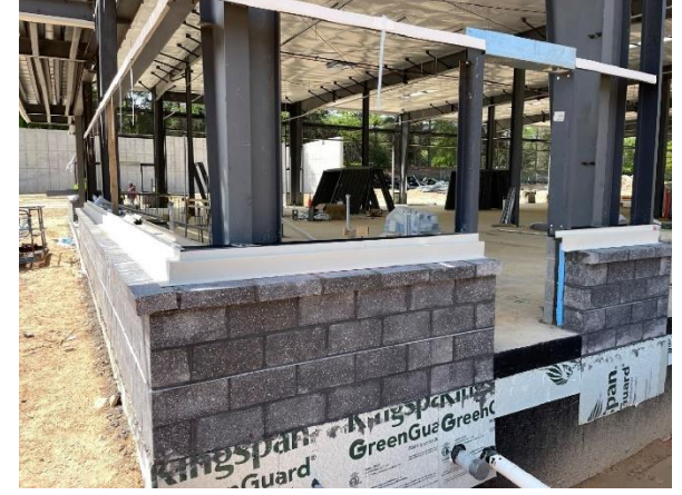
Exterior ground face CMU.
