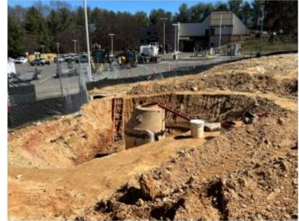
Installing manhole near a fuel station
