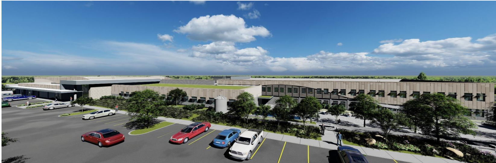
Building 1 – South Façade Front Elevation
