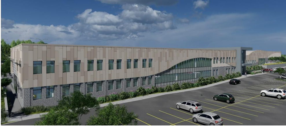
Building 1 – North Façade
