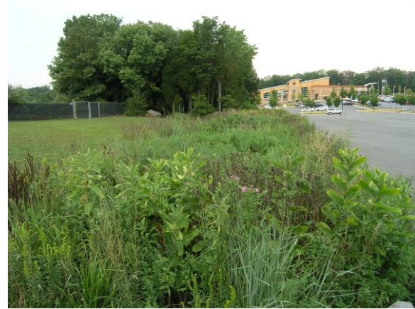
Figure 4-8: Vegetated swale (Source: Fairfax County)
