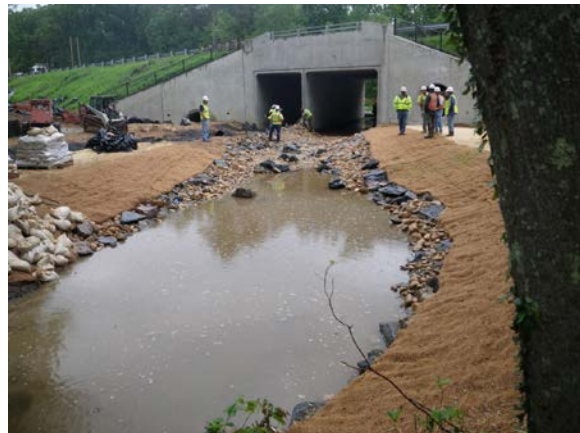
Figure 4-16: New replacement culvert (Source: KCI)
