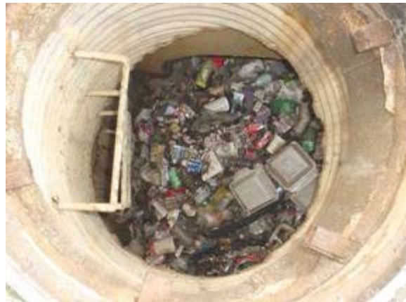
Figure 4-28: Catch basin (Source: Fairfax County)
