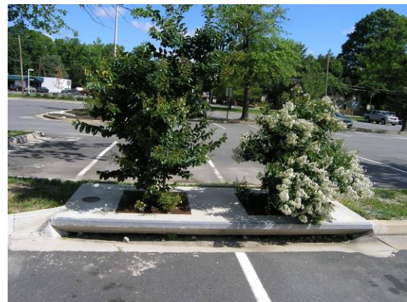
Figure 4-9: Tree box filter (Source: Fairfax County)
