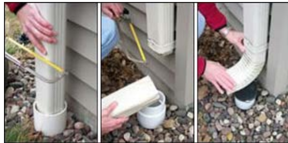
Figure 4-20: Disconnecting a downspout (Source: City of Toronto)
