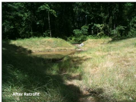
Figure 4-17: Outfall improvement (Source: Fairfax County)
