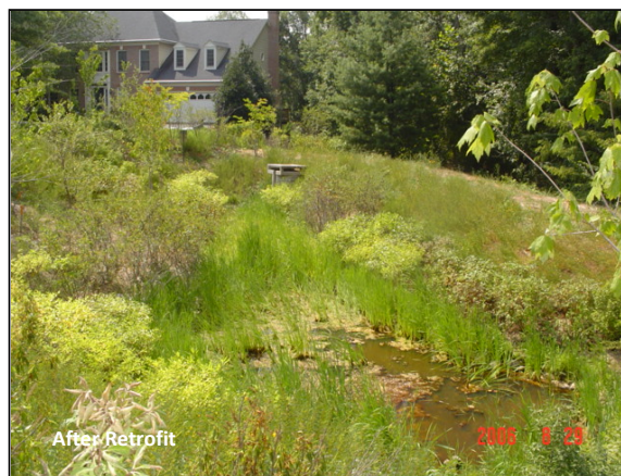
Figure 4-3: Stormwater dry pond retrofit (Source: Fairfax County)
