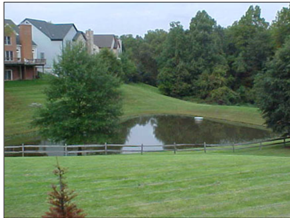
Figure 4-2: Stormwater Management wet pond (Source: Fairfax County)
