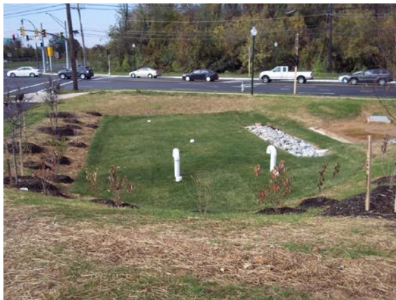
Figure 4-11: Sand filter along MD355 (Source: KCI)
