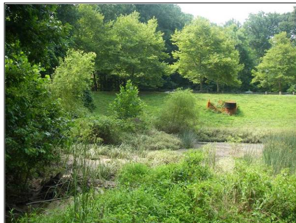
Figure 4-1: Engineered stormwater wetland (Source: Fairfax County)
