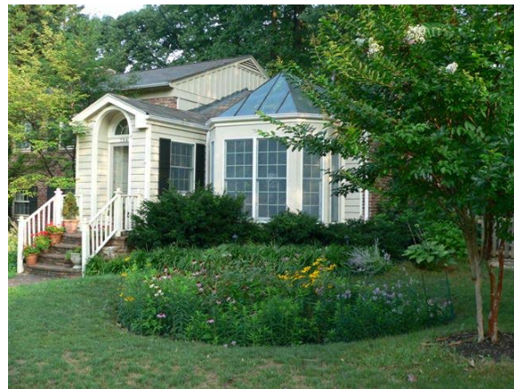
Figure 4-12: Residential rain garden (Source: Fairfax County)
