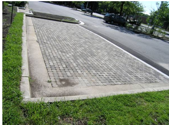
Figure 4-21: Permeable pavement blocks in a parking lot (Source: Fairfax County)
