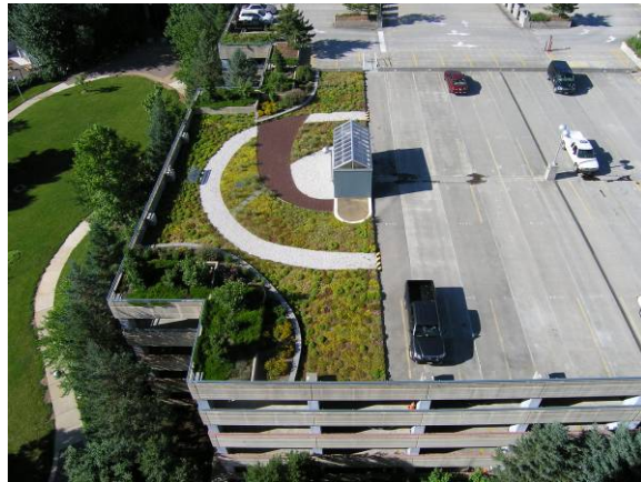
Figure 4-10: Green roof on a parking building (Source: Fairfax County)
