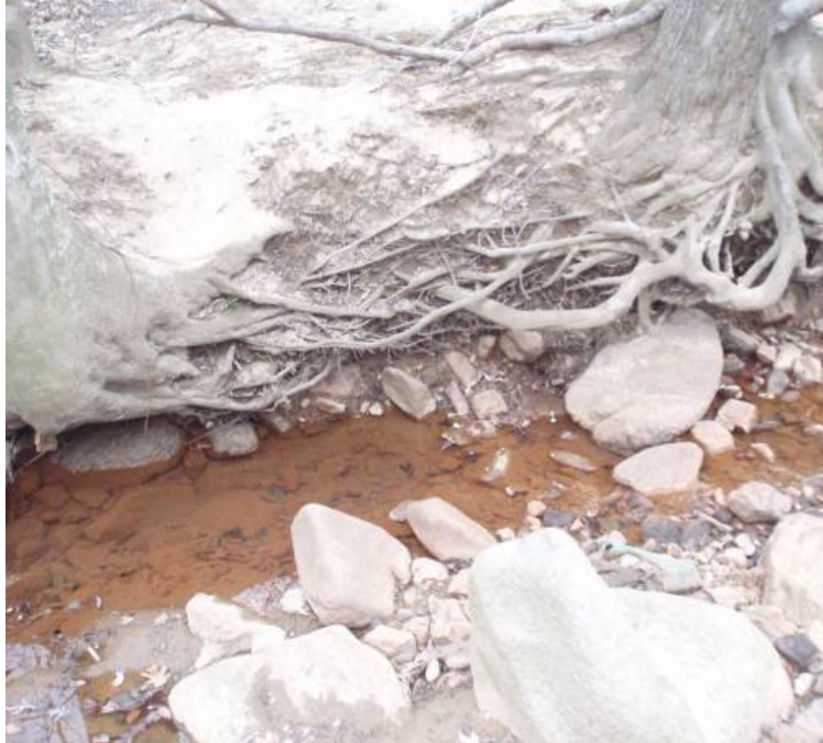
Site photo: Eroded channel
