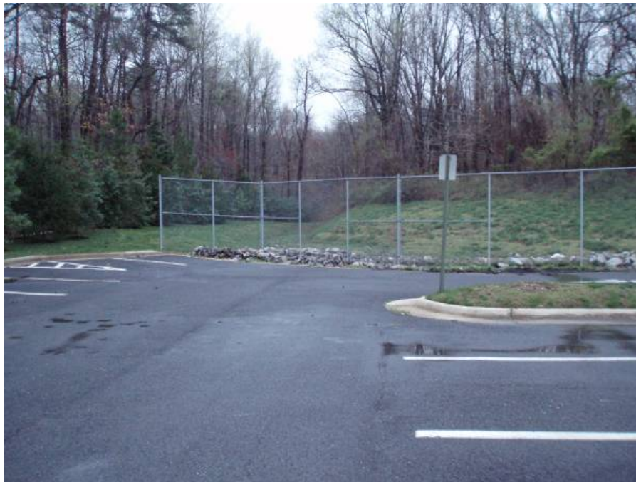
Site photo: Parking lot and bioretention facility location.
