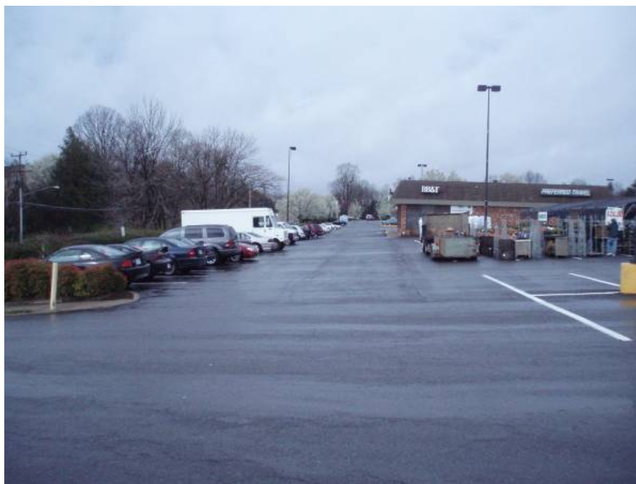
Site photo: Parking lot runoff could be treated by replacing end parking spaces with a bioretention filter.
