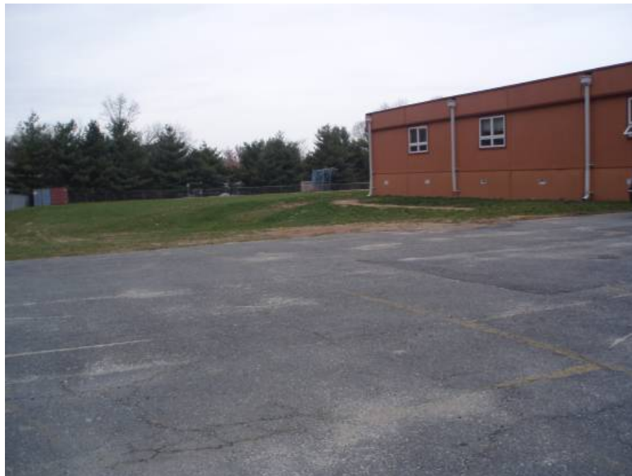
Site photo: Proposed location for a bioretention area to capture and treat parking lot runoff.
