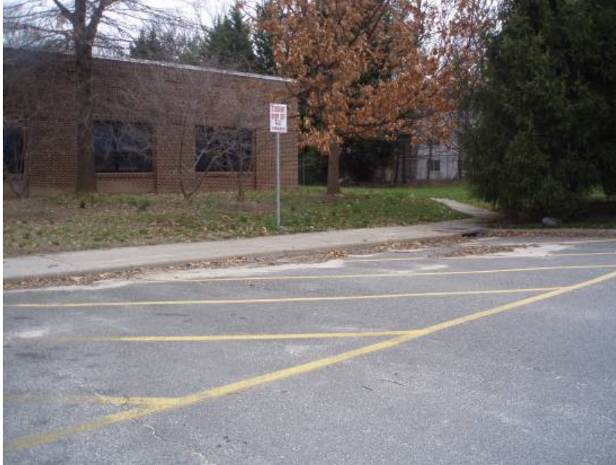
Site photo: Proposed location for a tree box filter to capture and treat parking lot runoff.
