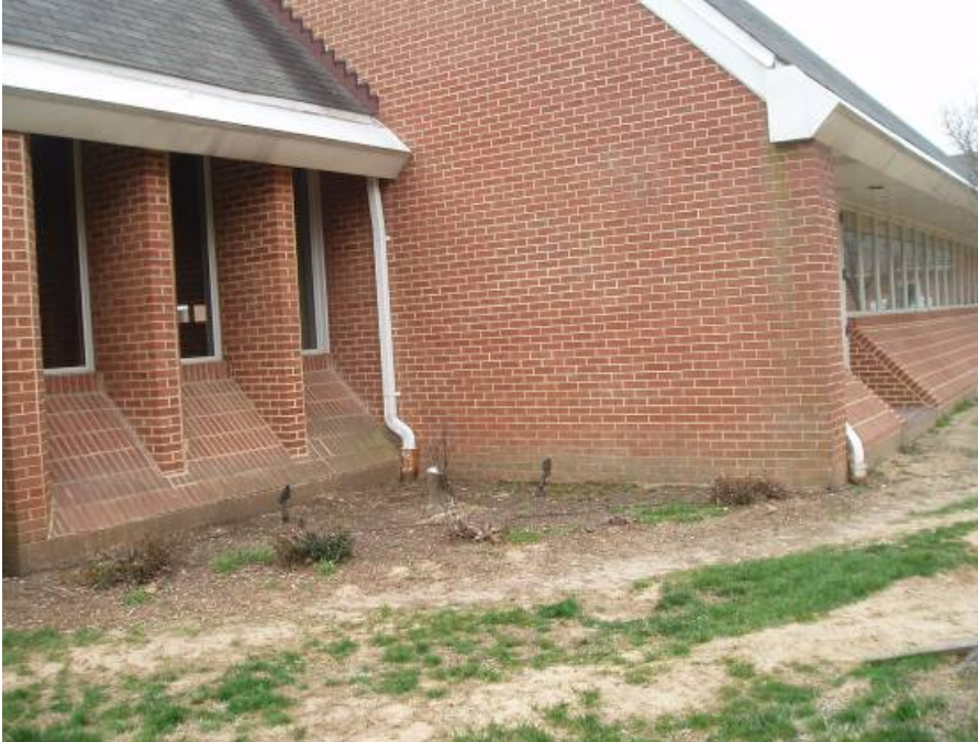
Site photo: Connected downspouts at the church for project AC9547A
