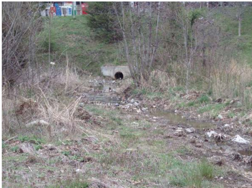
Site photo: Outfall to be treated by bioretention facility.
