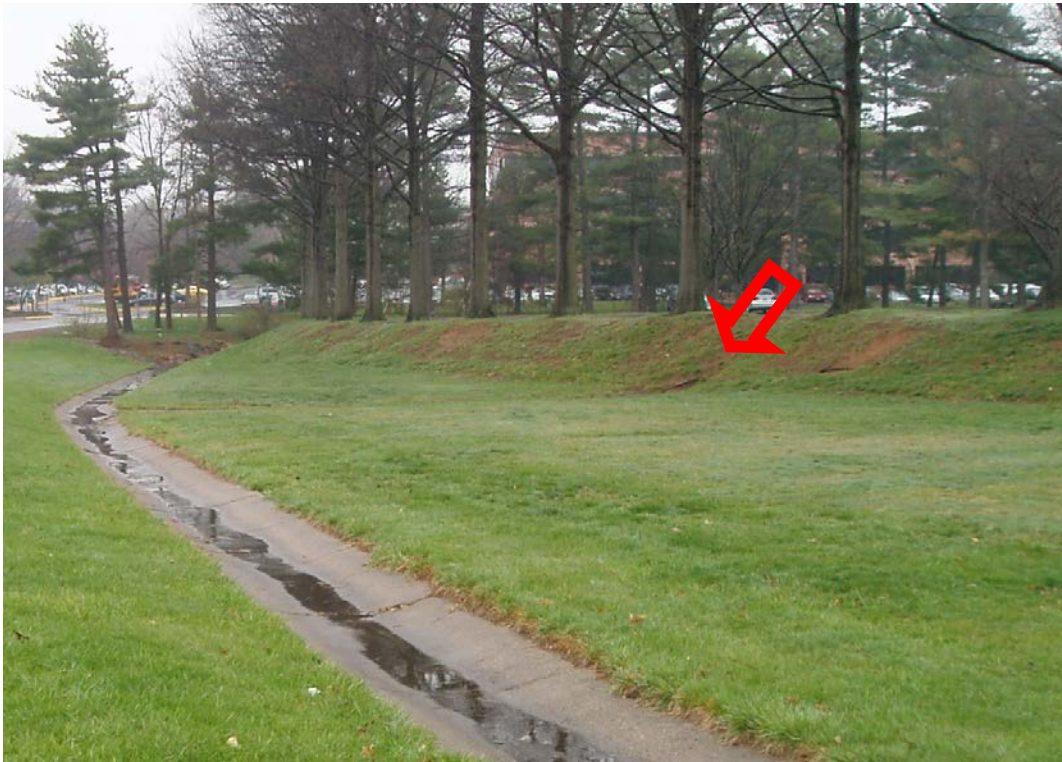
Site photo: One of three bioretention sites, at pond inflow as indicated.
