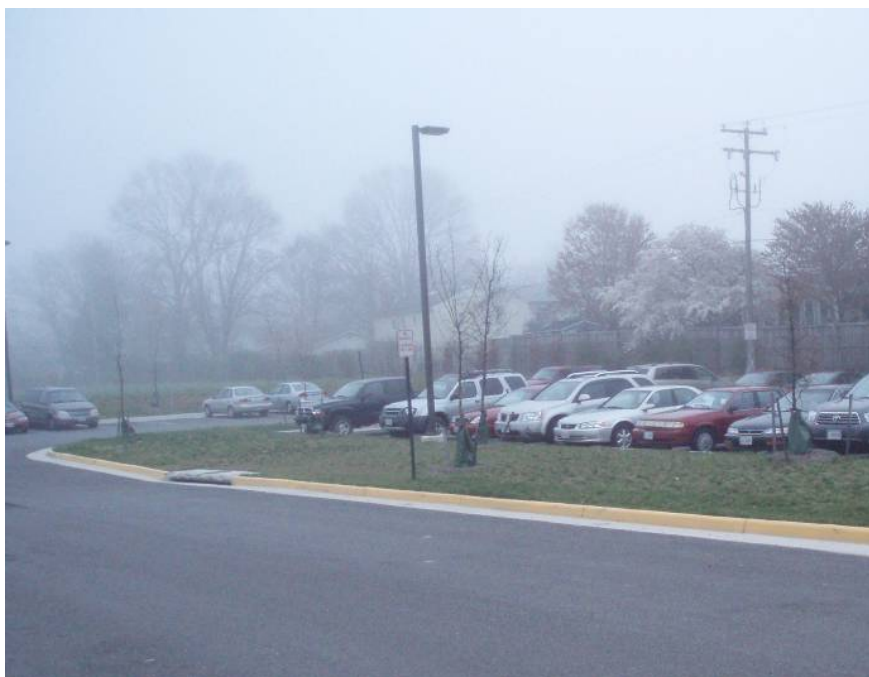
Site photo: Proposed location of one tree box filter adjacent to storm drain inlet in parking median.
