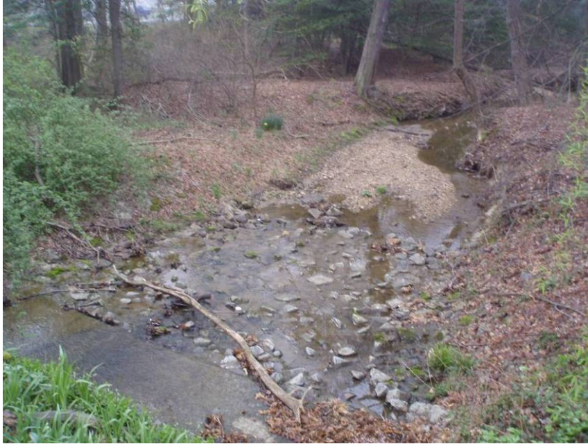
Site Photo: Downstream Floodplain of Culvert
