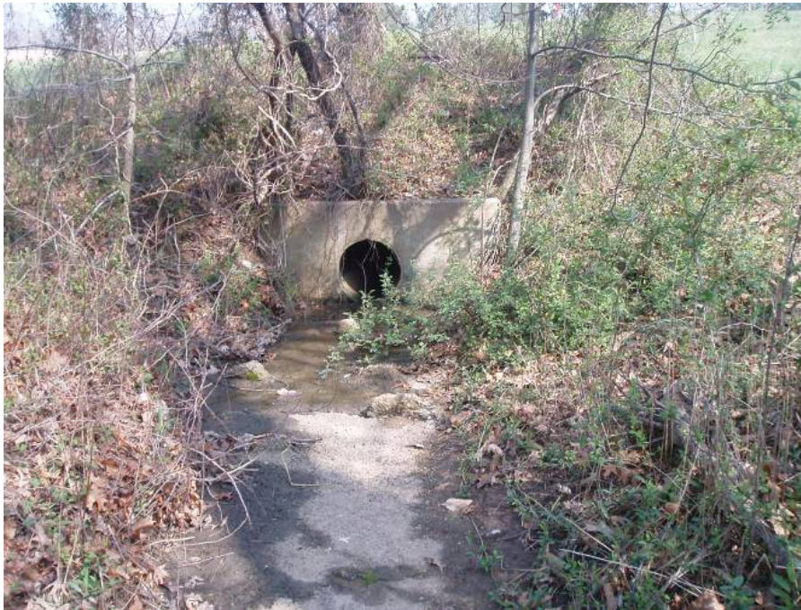
Site photo: Existing outfall on project site.
