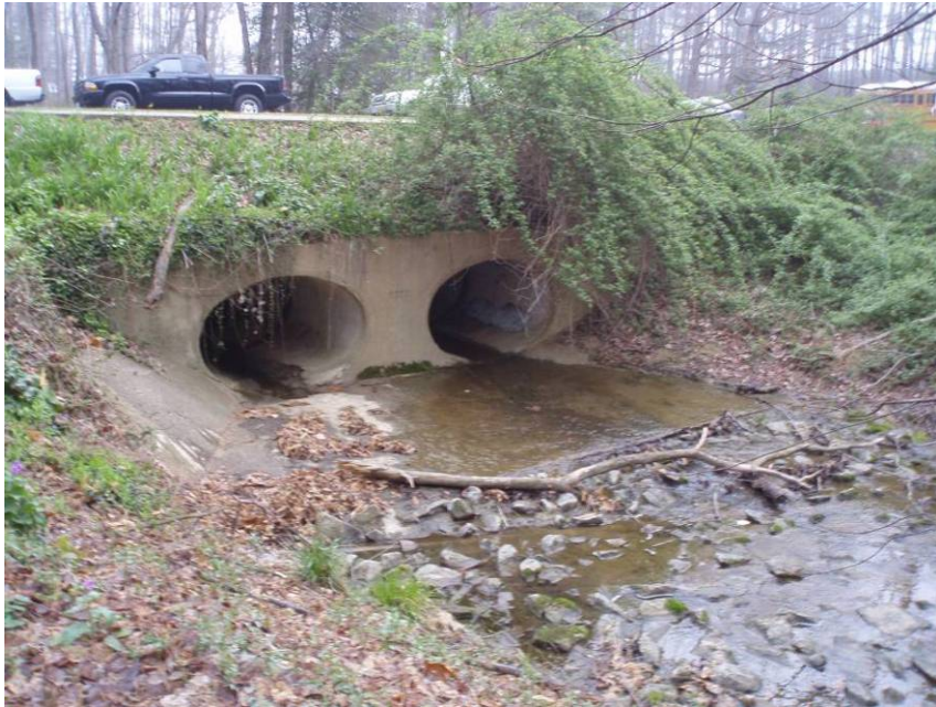
Site Photo: Existing Culvert
