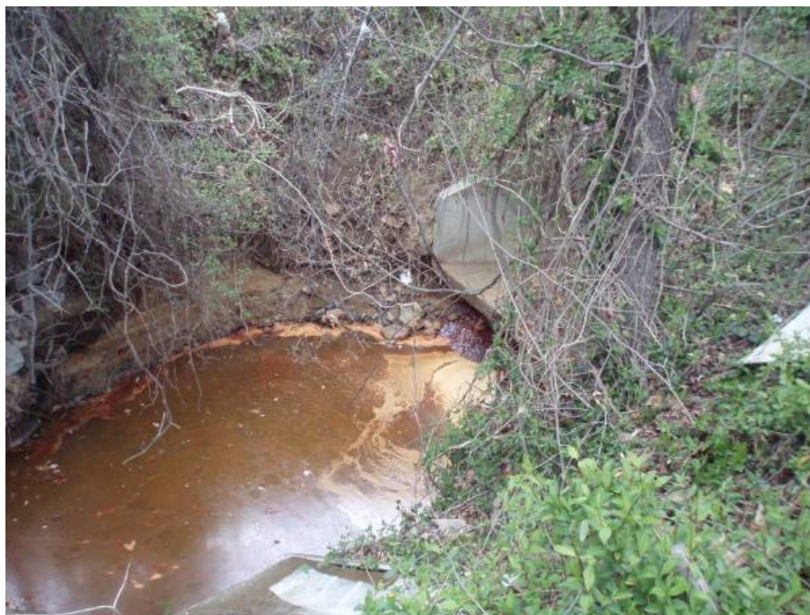
Site photo: Outfall to existing channel
