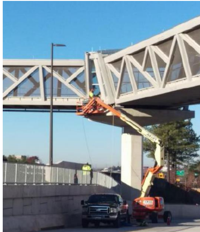
Finishing Trim on Reston N Ped Bridge
